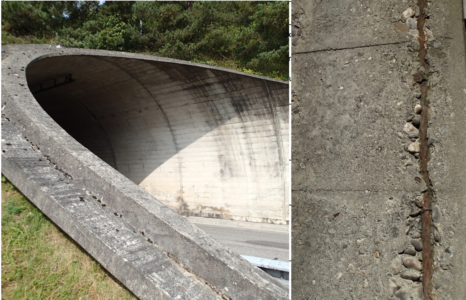
Example of very low cover depth, which should not happen
